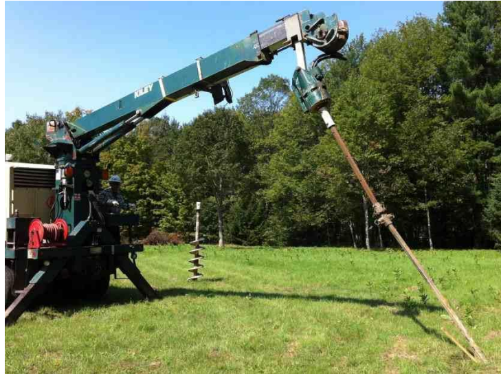
Figure 4.1 – Digger truck installing screw type anchors
