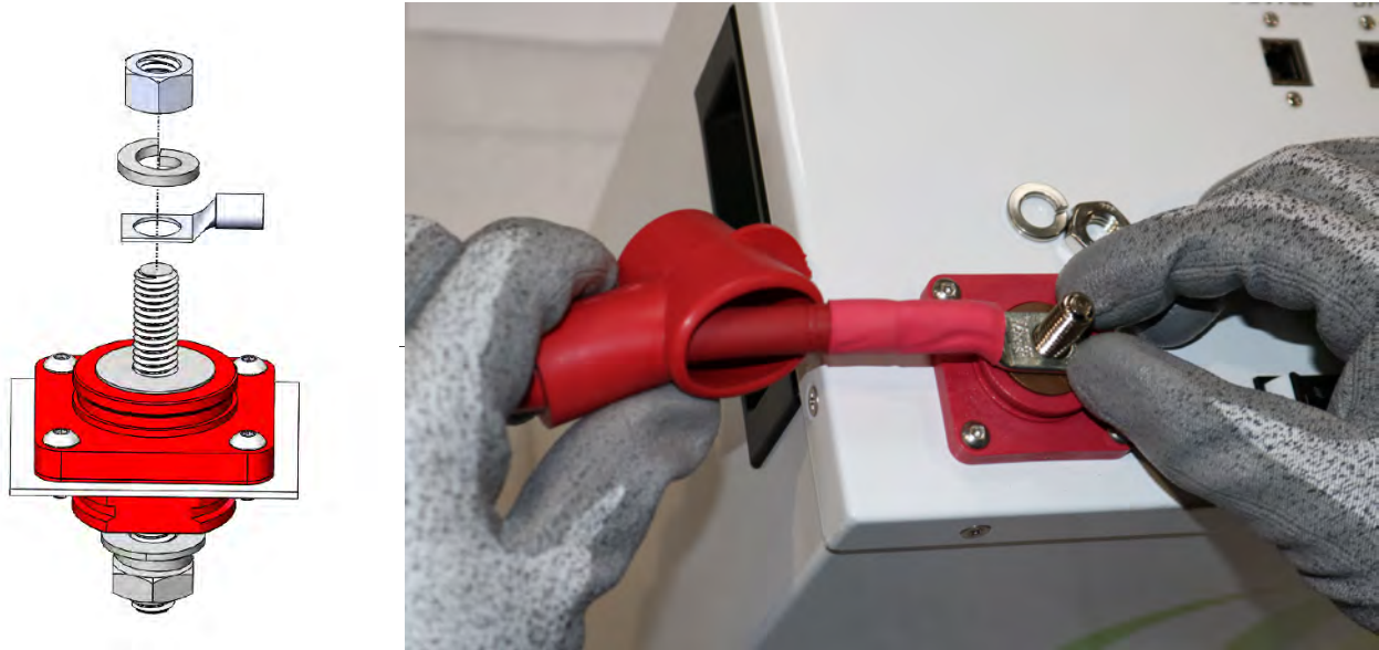
Figure 7.0 – Cable Lug Wiring onto AmpliPHI Threaded Stud
